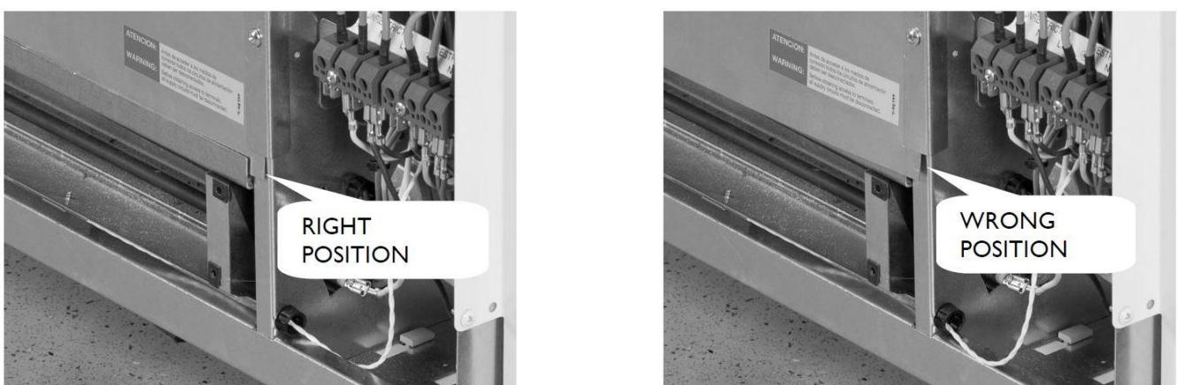
14. Replace the front panel. When refitting the exterior front panel, align the 2 metal upper pegs on the heater with holes in the exterior panel. Push the top up into place and push the bottom in, then refit the screws.
