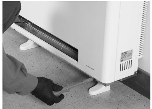
7.- Wire correctly the heater connecting Line, Neutral and Earth in the corresponding screw of the connection block. Tighten properly the connection block screws. Do not leave any remaining wire inside the heater.
